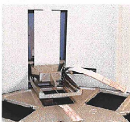
Figure 31 Both transport locks refitted
